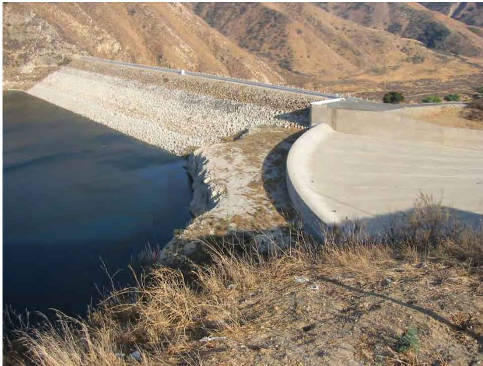
Figure 5-7. Santa Felicia Dam, looking downstream. (Photo by Stillwater Sciences)
