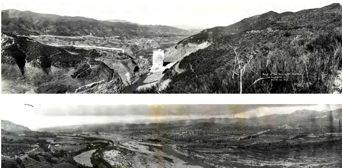
Figure 5-8. The remains of the Saint Francis Dam after collapsing just before midnight on March 12, 1928, in the San Francisquito subwatershed (above). Below, a downstream view of the mainstem Santa Clara River near Santa Paula Creek, the day after the Saint Francis Dam break flood. Photos courtesy of the Ventura County Watershed Protection District.
