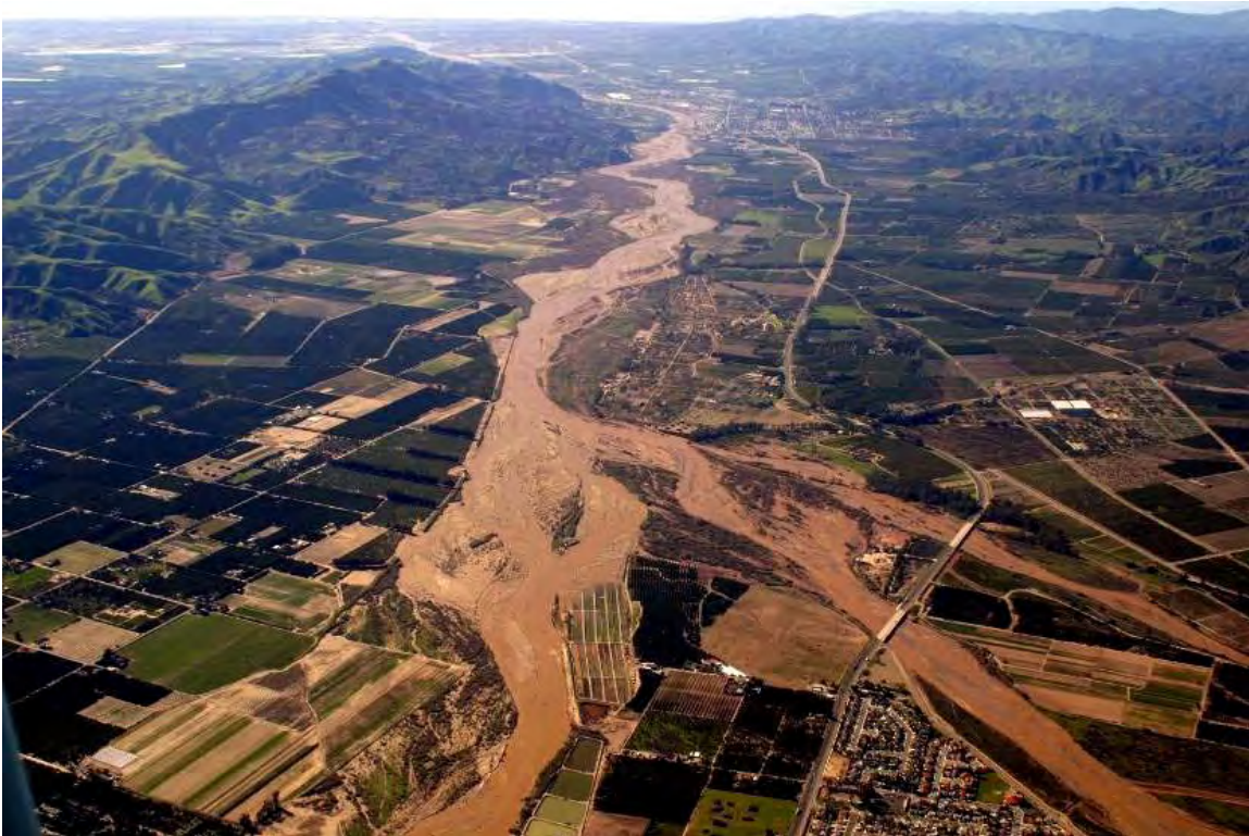
Figure 5-13. Westward, downstream view of the Sespe Creek confluence (two channels entering from right) following the January 2005 flood. South Mountain is in the upper left of photo. (Photo courtesy of the California Coastal Conservancy)
