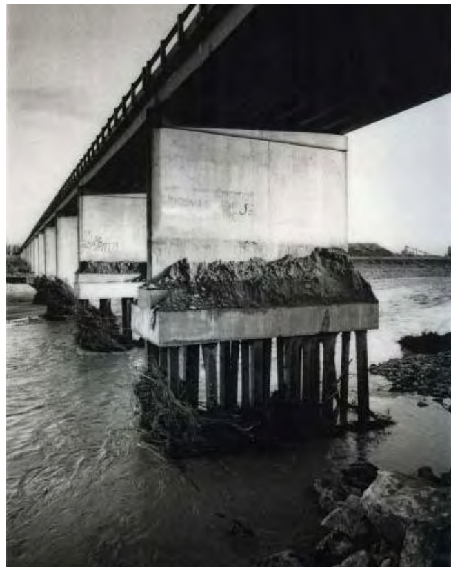
Figure 5-10. Undercutting of the Highway 118 bridge over the Santa Clara River as a result of incision following the 1969 floods. (Photo courtesy of the Ventura County Watershed Protection District)
